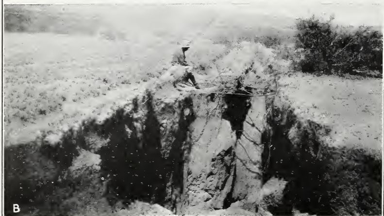
A.—Destructive erosion started in a cattle bedding ground in the arid Southwest. Even the grass roots can not hold the doomed land
